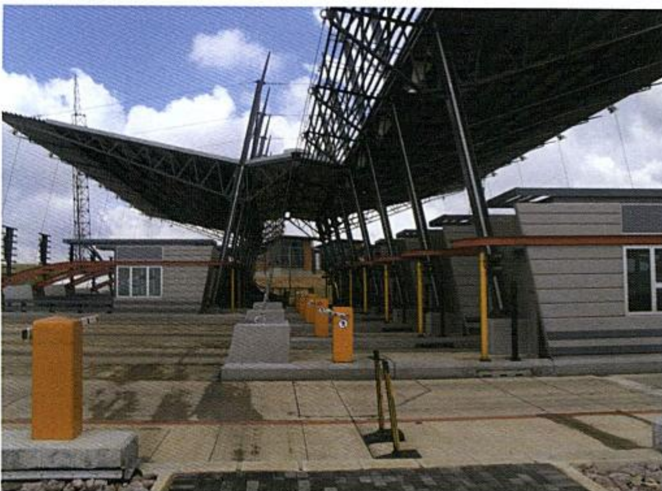
Diamond Hill Tollgate structure
